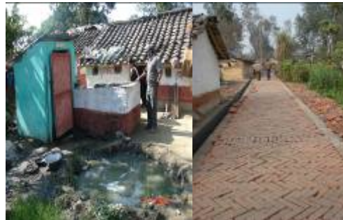
Figure 3: From left: A dirty water pond (before) and storm water drainage and paved road (now) have made the poor community able to have access to these services in Sangam tole.
