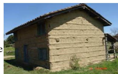
Fig. 1: Semi- permanent house built with Wooden frames, mud and tiles (a Traditional house slightly modified windows).
