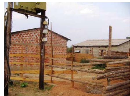
Fig 3: Similar design and construction methods using different building materials; clay and concrete blocks on the left and right respectively (source: author 2005)
