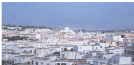
General view showing architectural characteristics of the quarter
