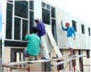
boards are being screwed
