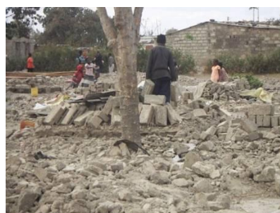
Figure 7: fully demolished house
