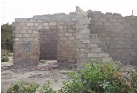
Figure 6: partly demolished house
