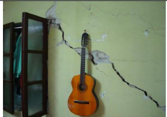
Inside a room of apartment building I2, Thanh Cong 2, Hanoi (Dothi.net 2008/1/9)
