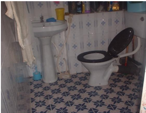
Figure 1: Altered bathroom after breaking the middle wall
