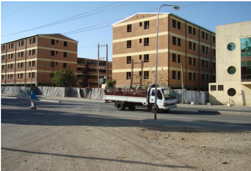
Figure 1. New condominiums with shops on the ground floor on a main Street
