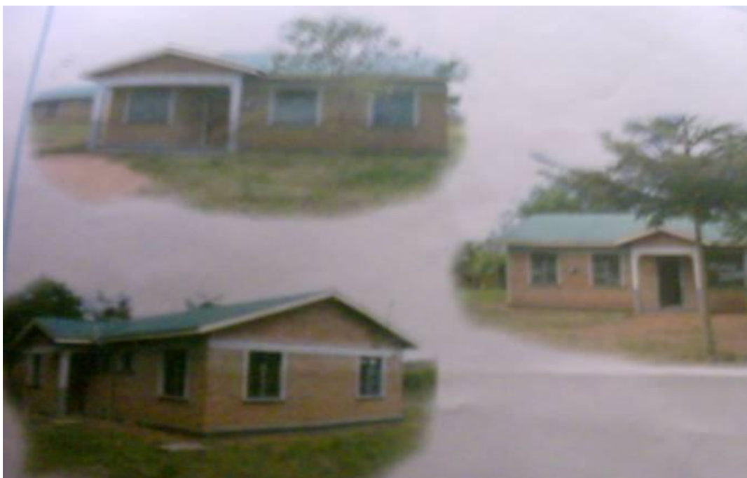
One of low cost houses built by PPF in Kisesa area, in Mwanza City
