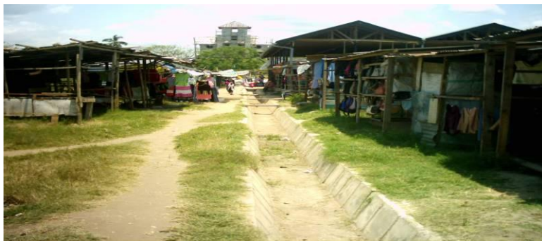
Improved market by Kinondoni Municipal Council with drainage channel, plenty of informal business around and waste blocking the drainage channel.
