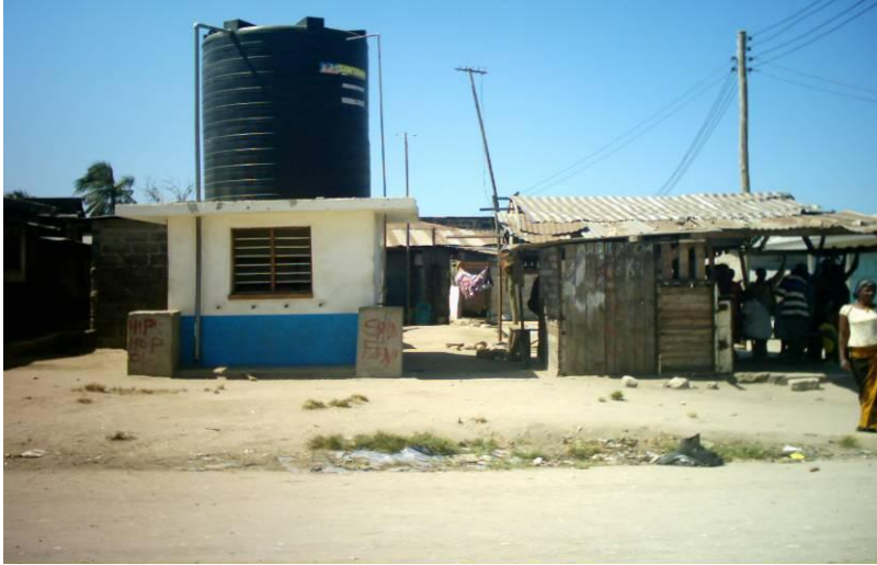
Communal water storage tank/ kiosk serving the community at affordable cost.
