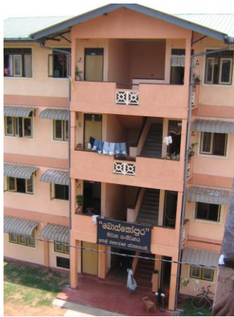
(Fig 5 –Common stairway lobby as drying yard)
