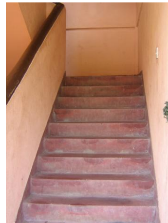
(Fig 6 –Covered Stairway –
