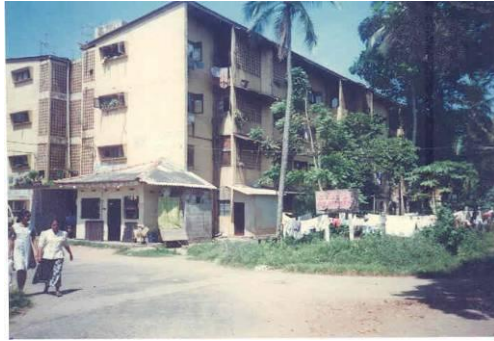
Fig 1: Exterior View of the Apartment
