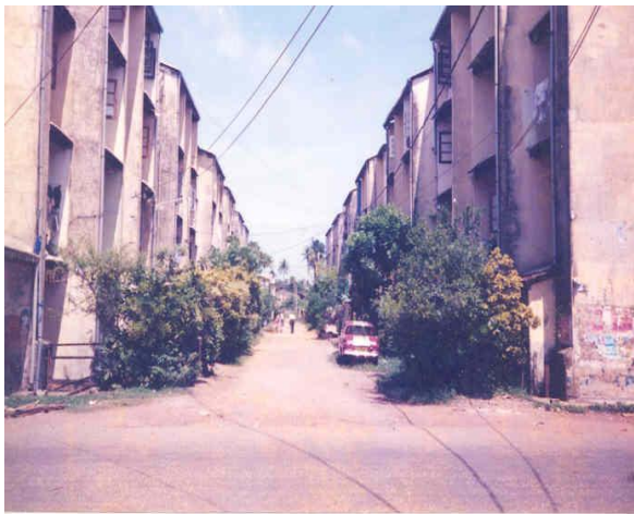
Fig 3: Exterior view blocks on either side of the road apartment
