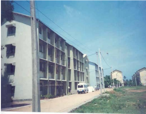
Fig 5: Exterior view of the apartment
