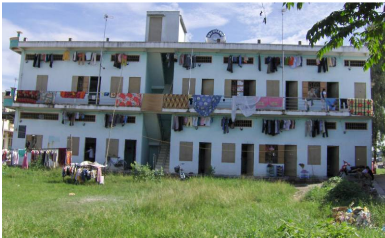
Figure 5: Renting block for workers built illegally by landowner (Source E-City, 2008)
