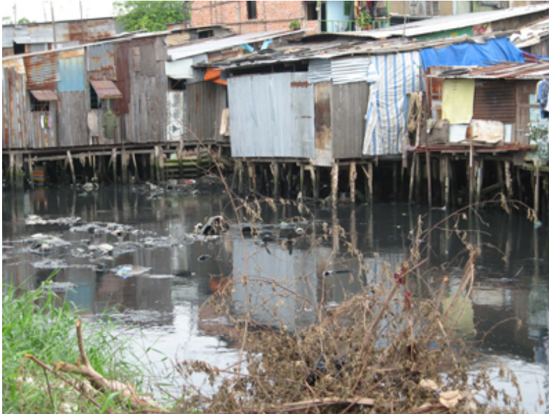
Figure 6: Slump area in Ho Chi Minh City (Source E-City, 2008)
