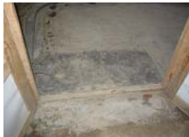
Fig 13: Kerb ramp at the threshold point of the door
