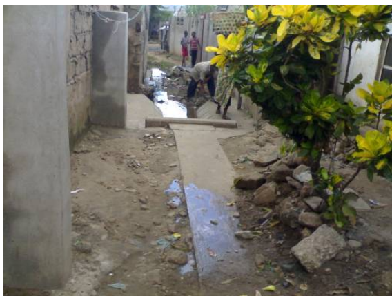
Poor drainage facilities
