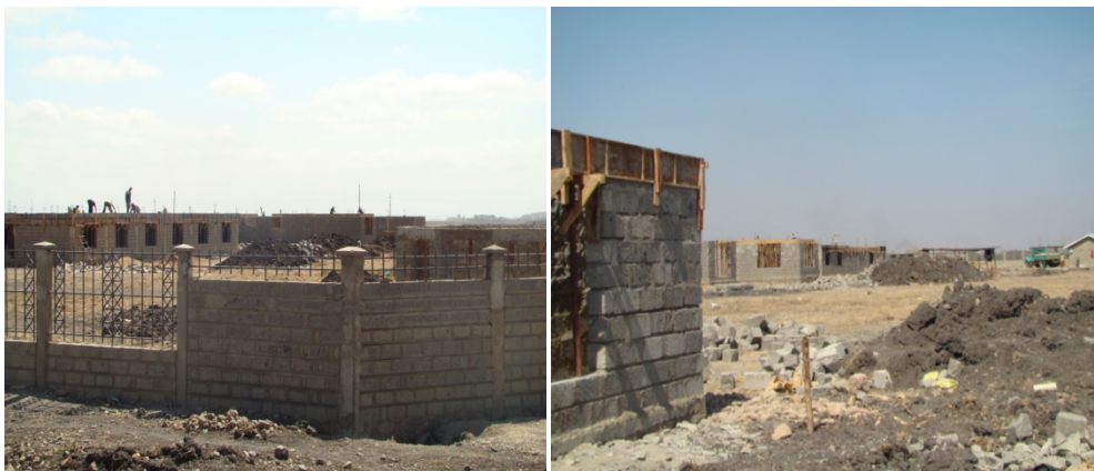
The ABT centre seen from the road.
