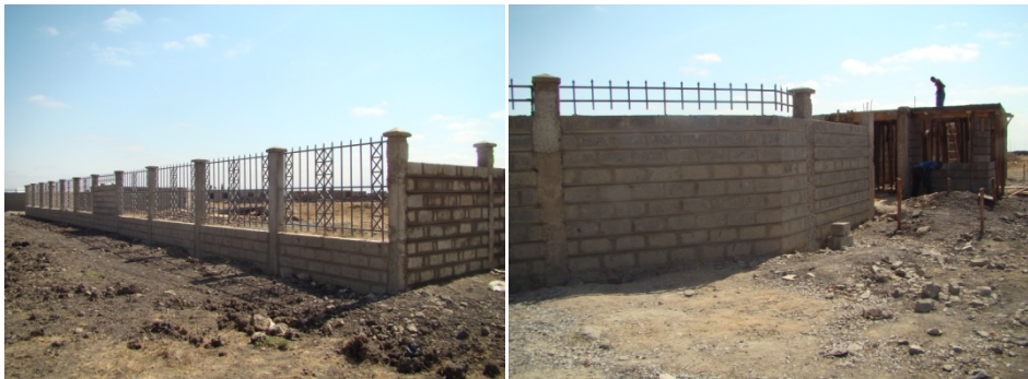
The perimeter wall and part of the gate house under construction
