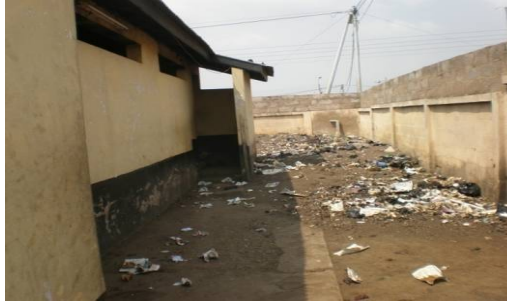
Plate 5: Poor Surroundings of a Public Toilet Facility
