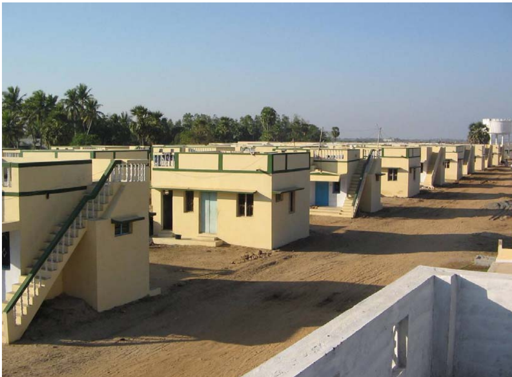
View of Reconstructed Poombuhar Shelters
