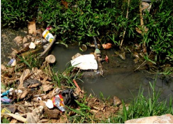
Picture 2: Water pipe going through contaminated water.
