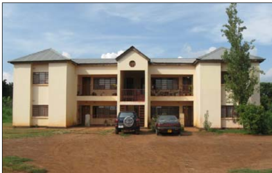
Figure 4 Two Storey Teachers Block of Flats at David Kaunda Technical High School in Lusaka District. Picture by Author, January 2010
