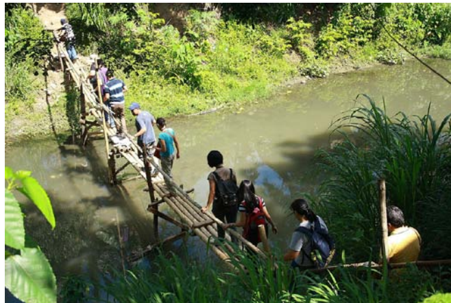
Figure 2. Bamboo make-shift bridge of Matina Crossing community, Davao
