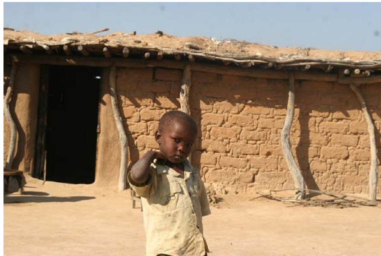
Typical rural house using traditional building materials, such as, mudblocks and pole
