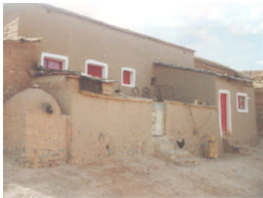
Improved adobe housing in Tupiza.
