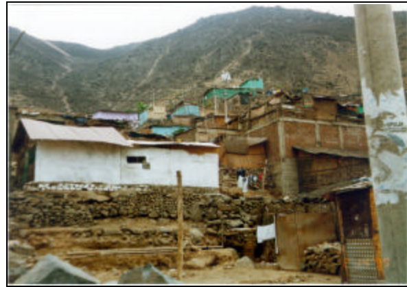
Figure 5: Foundations called "Pircas", used by the precarious houses in the settlement of Saul Cantoral.
