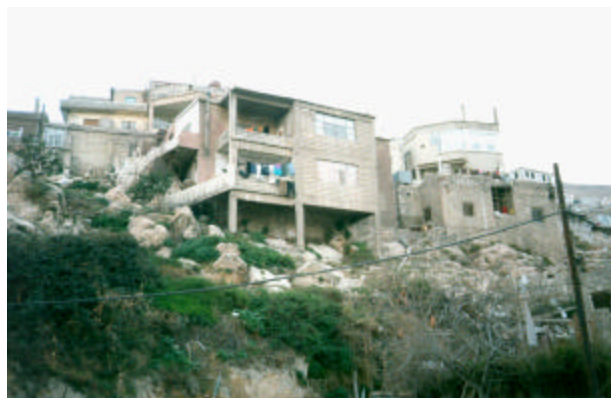
Figure no 3: it shows the illegal construction houses built by the people.
