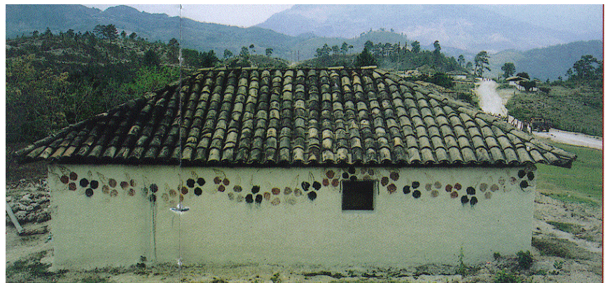
Painted adobe house
