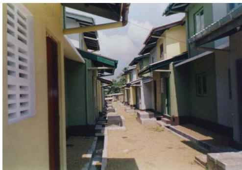
Fig 5 Facilitating of on-site infrastructure including roads, electricity, water supply, sewerage and waste water disposal so on. (Source: photo by author)
