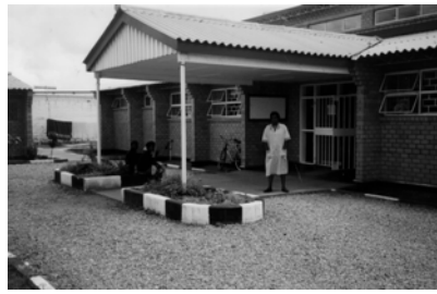
Photo 1: View of approach to the ward.
