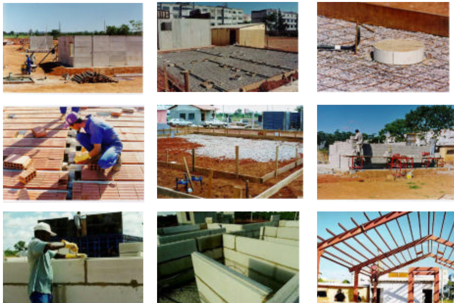
Figure 3: Examples of photos taken during the building process
