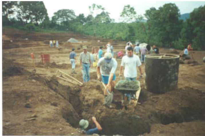
Figure 3: Construction phase: Construction of infrastructure in Nazareth Condominium
