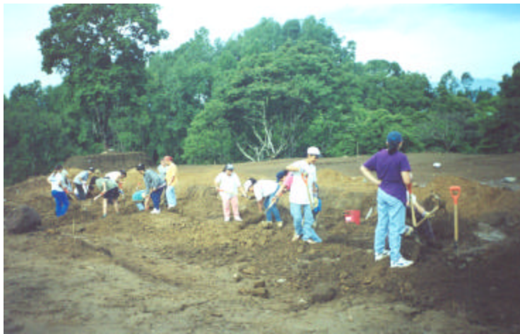
Figure 4: Self-help construction with mutual help in Nazareth Condominium.
