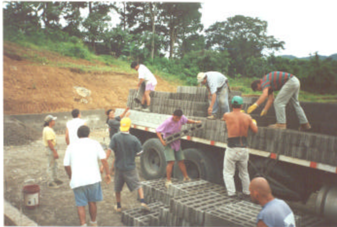
Figure 6: Construction material called "Super block" was used in construction of houses
