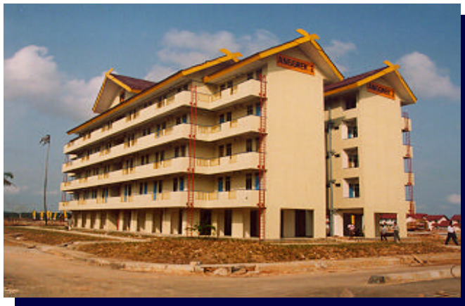
Figure 12: Multi-storey building for low income people, location: Cengkareng, Jakarta
