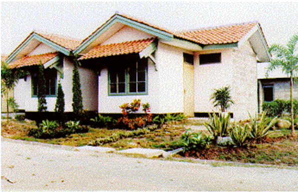
Figure 8: The middle-income house type 21/72 with clay tile roof in Driyorejo, Surabaya
