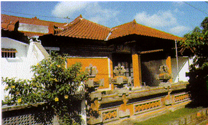
Figure 9: Sample of native cultured based house for middle and high-income people in Bali.
