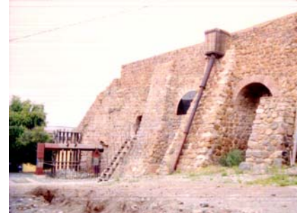
Figure 3. Molino del Rey (King’s Mill) in “La ribera” Picture: A. Balderrama 2005
