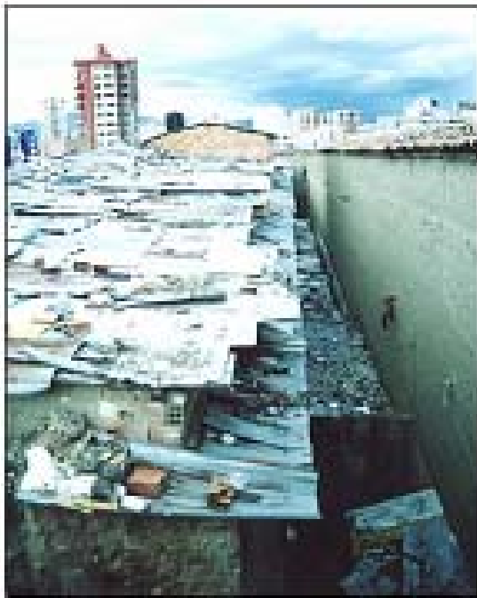
Figure 19. "Cells" on the roof
