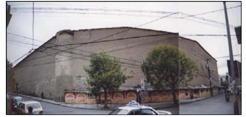
Figure 18 Kiosks attached to the back
