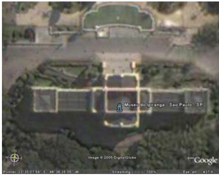
13 The building as seen from above
