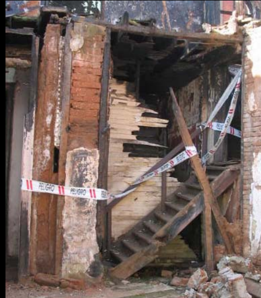
Foto N° 10: Present state image of tabiquería interior
