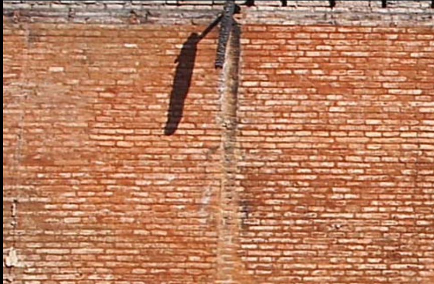
Foto N° 6. Beam Metallic Lintel, in vain of doors and windows Analysis Fire walls. The Severín building has two fire walls, one leaned to a structure by street Santiago Severín, which also was destroyed in the fire and other that it gives towards Santo Domingo street where at the moment inhabited constructions exist. The fire walls are of masonry and they are in good state as it is possible to be appreciated in the following photography's.
