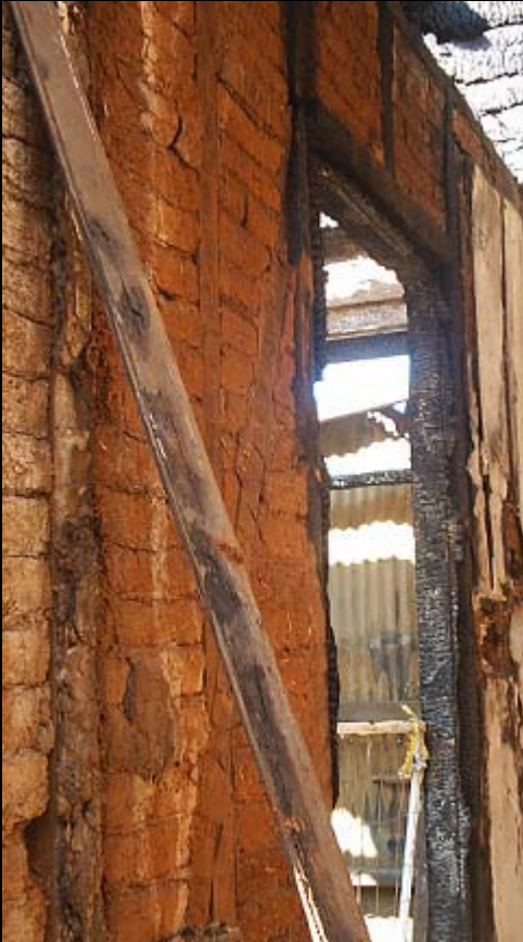
Photo N° 5 Present situation of the inner structure of the Building....
