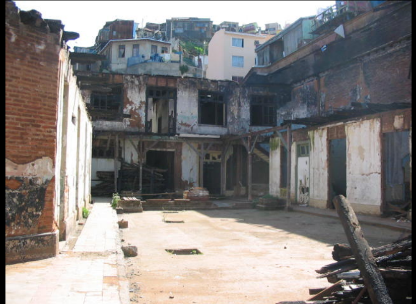
Photo N° 4 Present situation of the inner structure of the Building.
