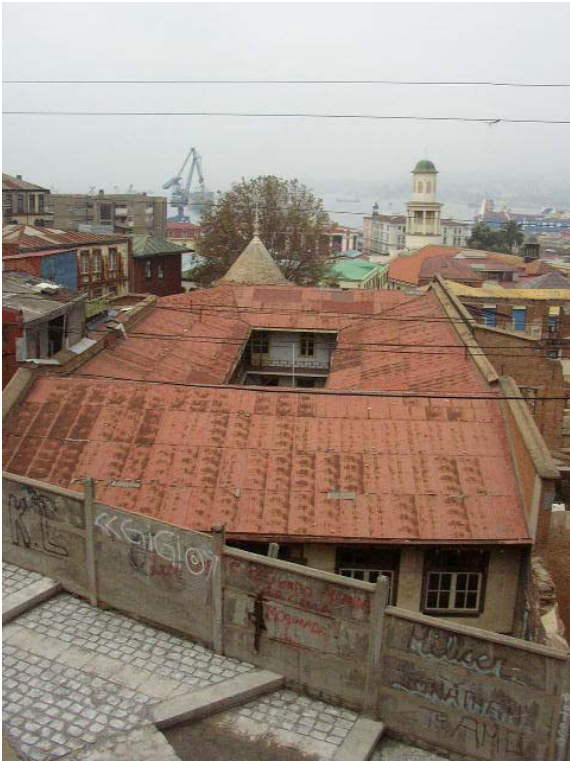
photo n°1 Roof of the building before the year 2003
