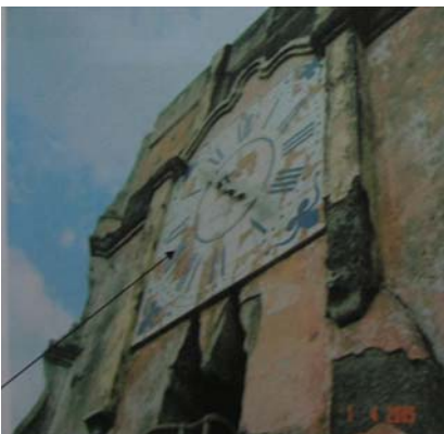
Fig. 24,26 “missing parts in element's shape”
