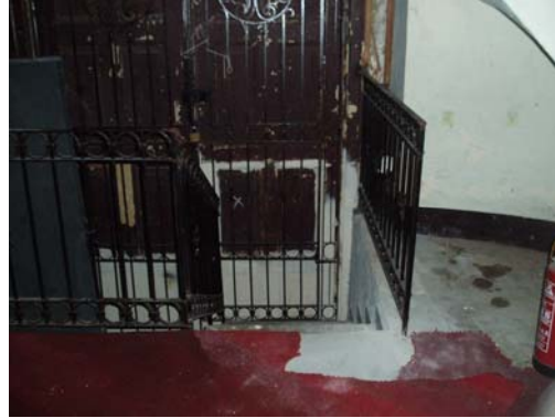
figure 100: Handicapped persons entrance
