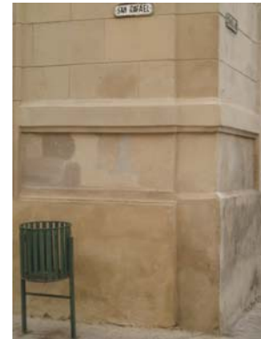
figure 68: Facade in restoration
