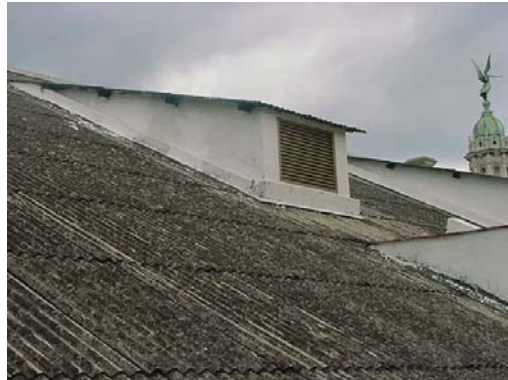
figure 61: Restored roof- asbestos tiles
