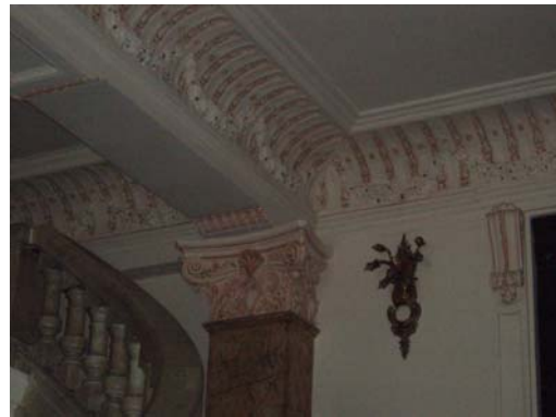
figure 27: Interiors walls- Lobby
