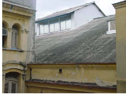
figure 18: Asbest tiles
