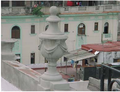
figure 65: Restored elements on the roof
