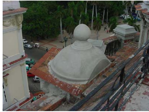
figure 66: Restored elements on the roof
