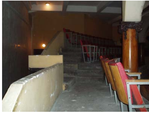
figure 38: Corridors, masonry walls
