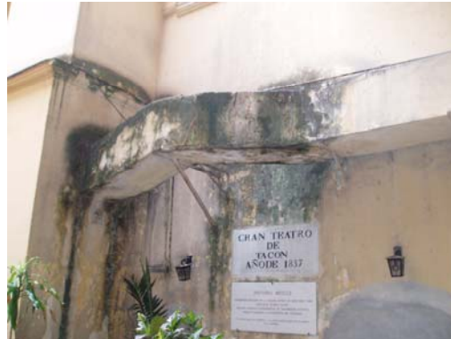
figure 45: Moisture surfaces
