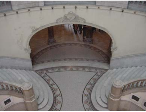
figure 22: Stair, Galician Center Lobby
