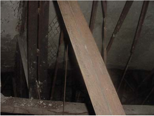
figure 43: Steel structure, good state
