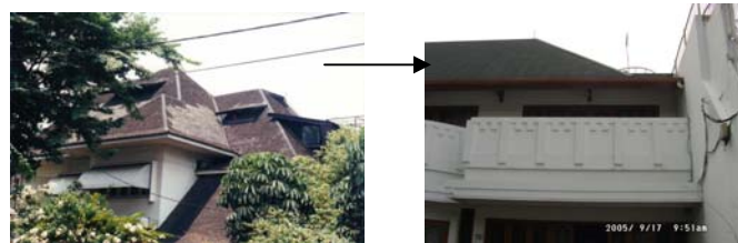
Picture 18: The old and new roof material.
