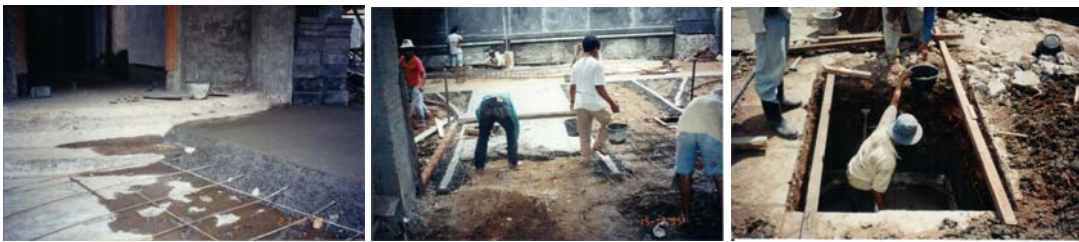
Picture 14: Floor construction and drainage ditch under car park.
