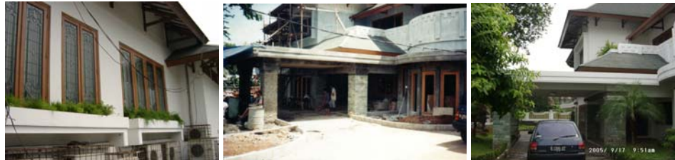
Picture 20: The outdoor units of air condition and the new car port.
