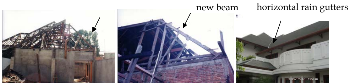
Picture 12: Roof construction process and the horizontal rain gutters.
