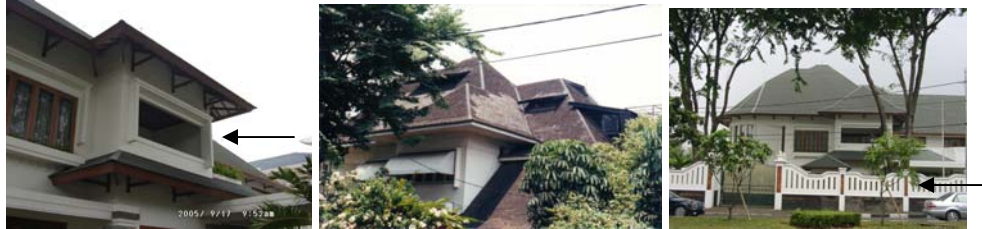
Picture 22: The new balcony and fence.
