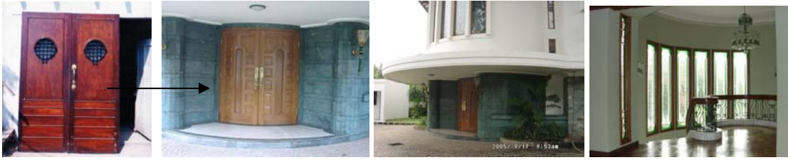
Picture 16: The old and new main entrance door and the art glass on window.
