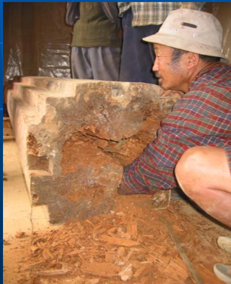
Examination of kachens and removal of the decayed heart wood.
