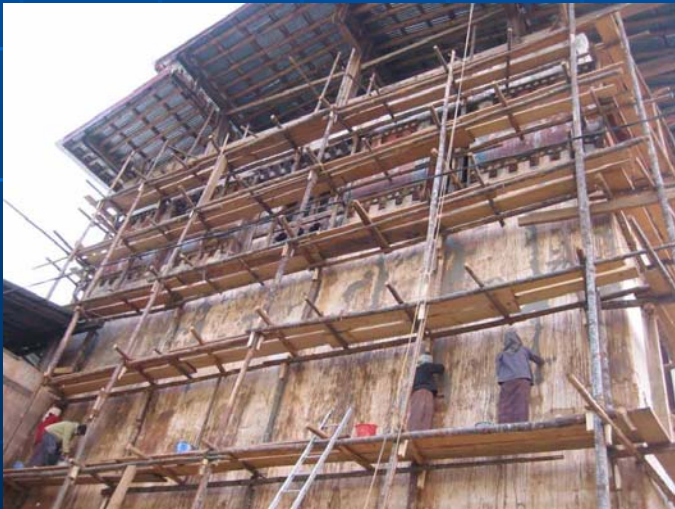
Repairing of cracks in the rammed earth walls
