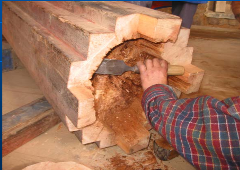
Examination of kachens and removal of the decayed heart wood.
