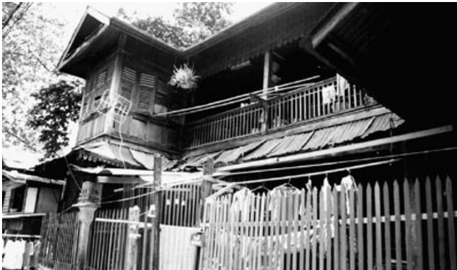
Fig.2 Photo of House in Mahakarn Fort Community
