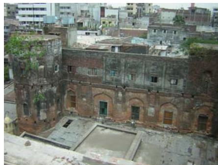
Fig. 16 New settlements, close to the South wing
