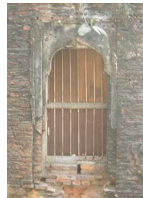
Fig. 43 Window from outside
