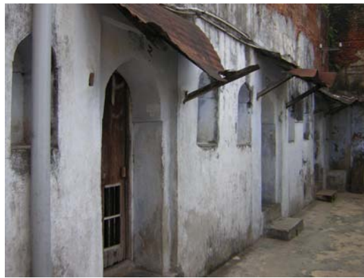
Fig. 42 New addition of door-shades at the terrace
