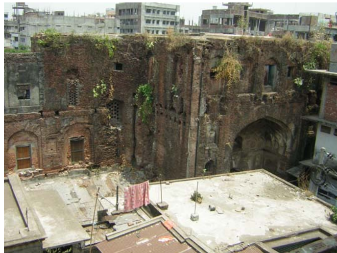
Fig. 20 Existing south wing
