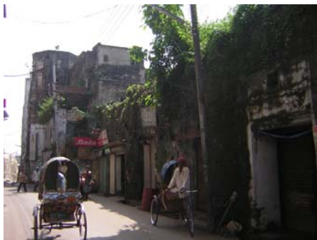
Fig. 13 East wing from the road
