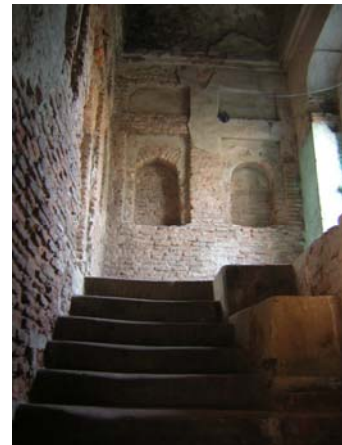
Fig. 36 plaster removed from wall
