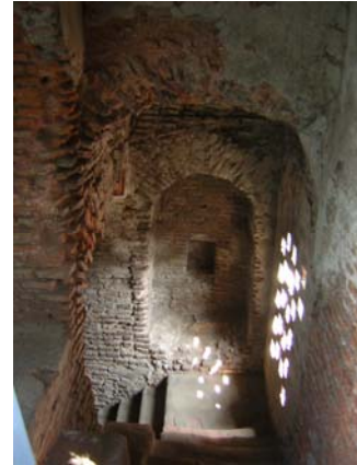
Fig. 30 Natural lighting inside staircase
