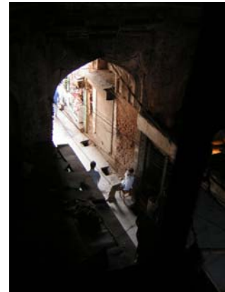
Fig. 3 Walkway through the existing entrance hall
