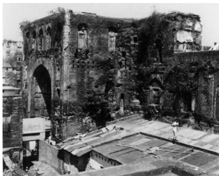
Fig.11 Entrance, south wing,1964
