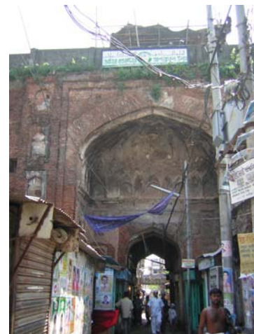
Fig. 21 existing entrance hall from north
