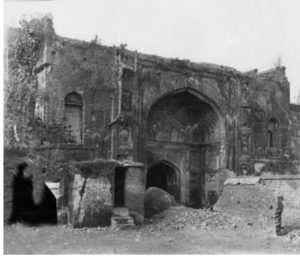
Fig.9 Entrance, south wing from the courtyard.1950
