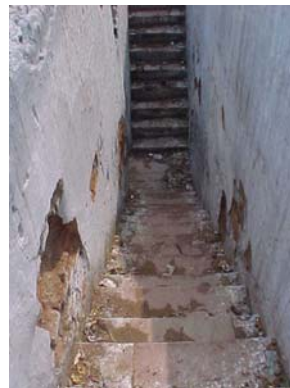
Staircase on the West side
