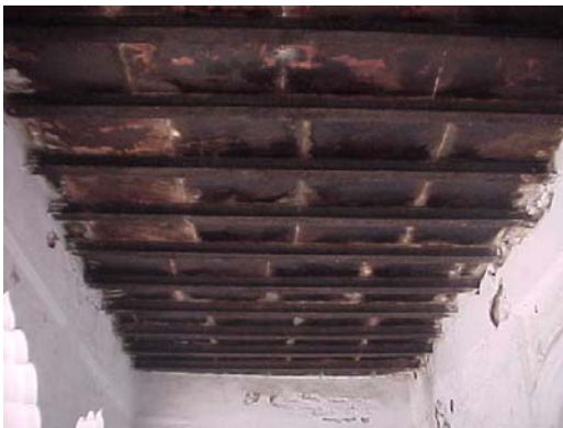
Roof pattern in some of the rooms
