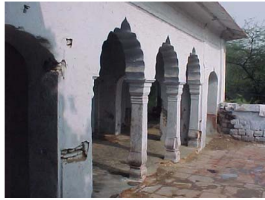
First floor structures
