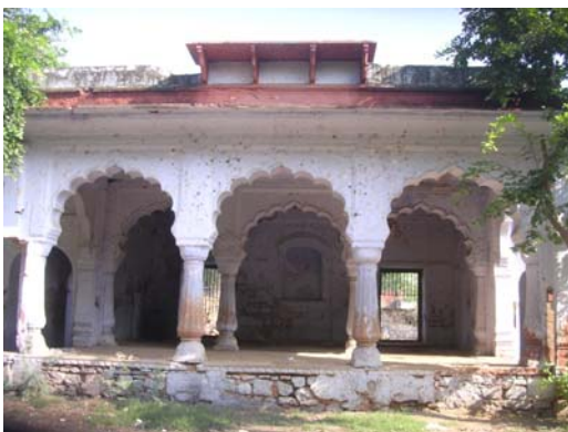
Chambers on north side of the site
