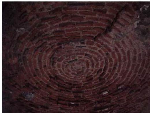
Roof in the North West corner chamber of the site
