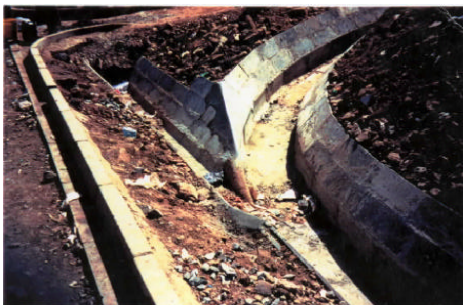
Basic storm-water drainage improvements
