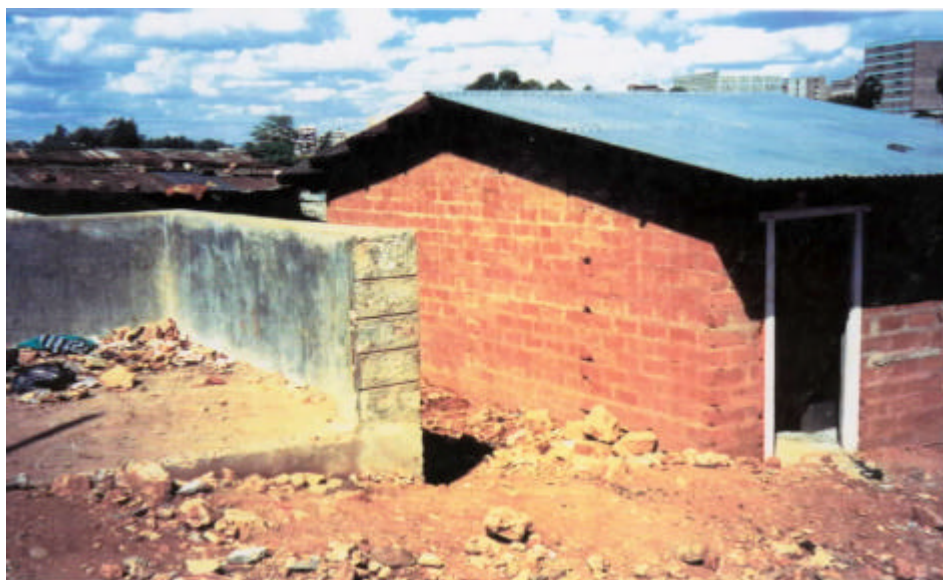
Wet core facility containing a toilet, shower and washing place
