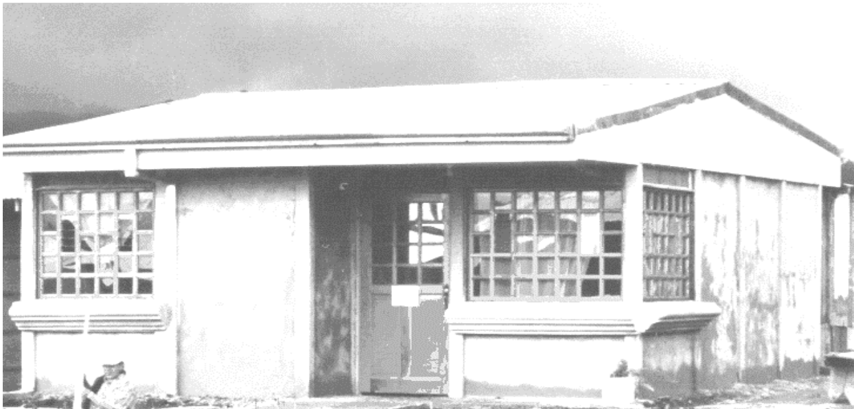
Figure # 2, Prefabricated House in Lagos de Lindora's Project
