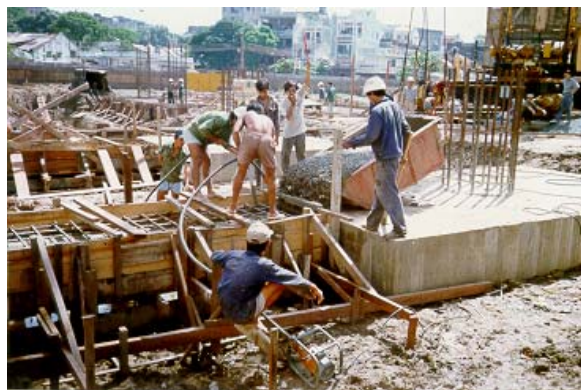
Casting Concrete on Site.
