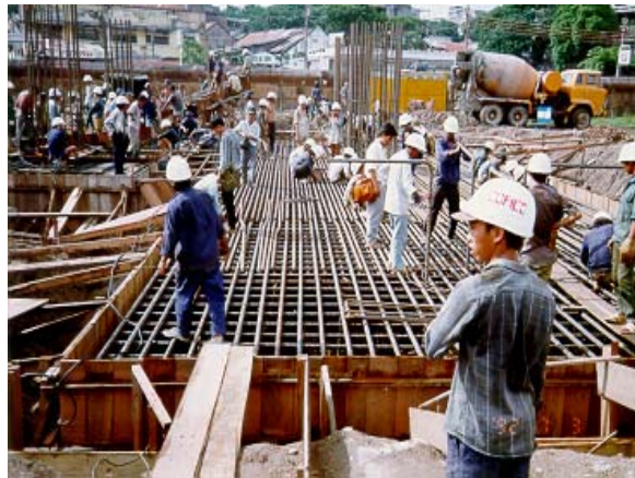
Installation of Rebars and Formworks
