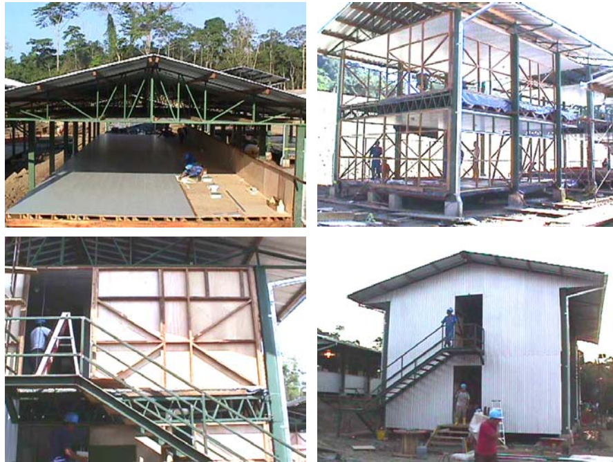
Figure 5: Different stages of construction
