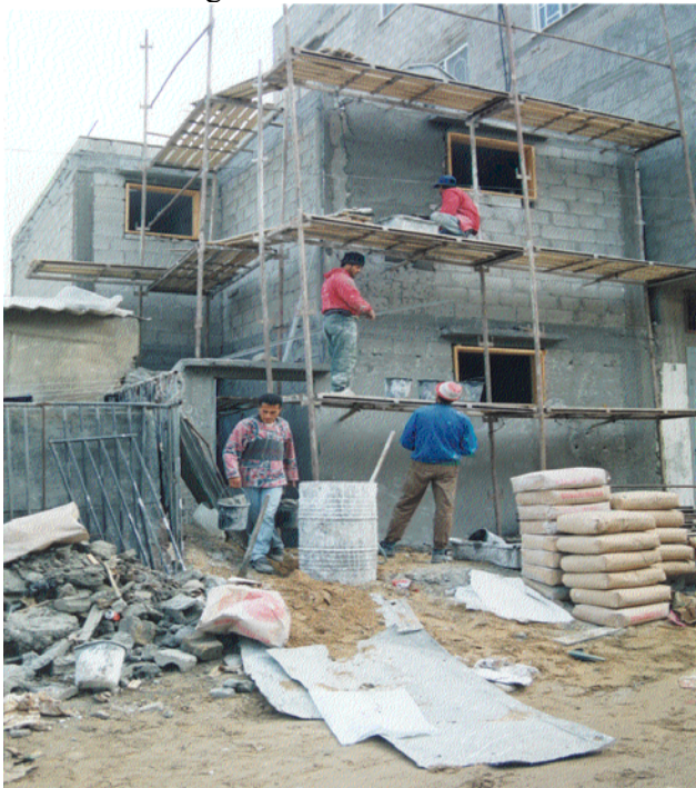
Shelter of two floors under construction, in beach camp, Palestine
