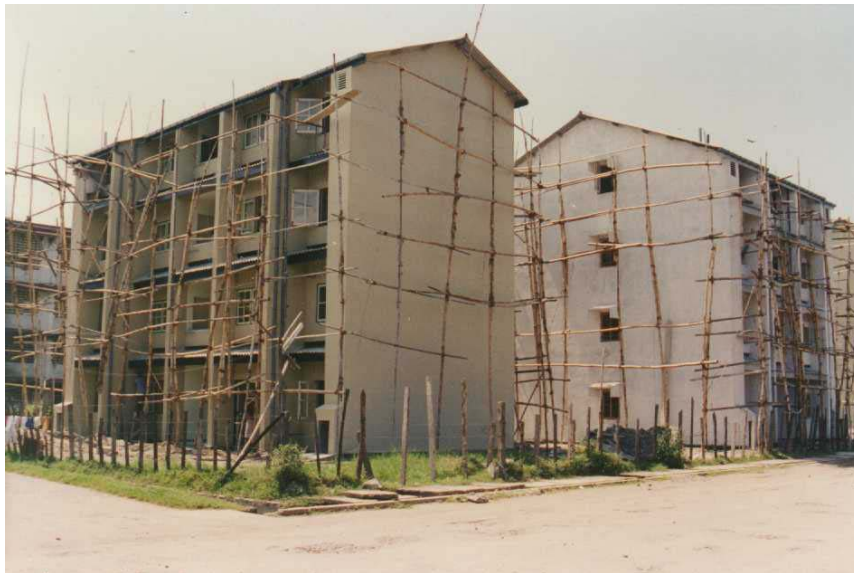
Four storey walk-ups in finishing stage
