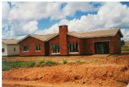
Completed High-income house.
