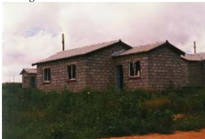
Low-income house under construction.
