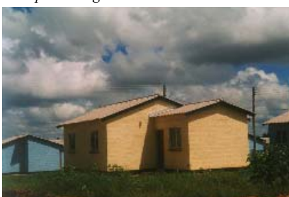
Completed Low-income house.
