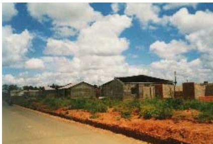
High-income house under construction.
